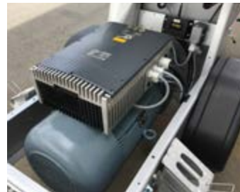
The 22 kW Electric motor
